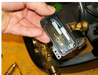
Check the pressure-switch switching capacity and continuity by using a multimeter.
