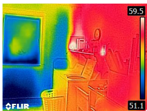
Uninsulated outside wall
