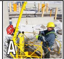
**IMPORTANT:** Make sure the lifeline cable or rope is positioned directly over the work area. Use only certified lifeline cable or rope, in perfect working condition, with appropriate specifications, including maximum leverage capabilities, for the intended use of the XTIRPA system.
