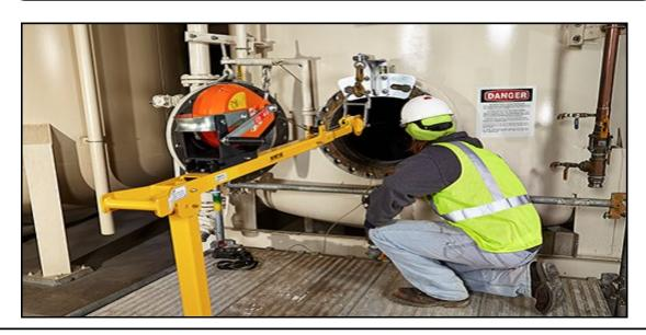
**IMPORTANT:** The connectors (EN 362) (hooks, carabiners, D-rings) must be able to support a weight of at least 5000lbf (22.2kN) for ANSI, CSA, OSHA and 12kN for EN-795:2012.
