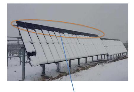
Vertical installation, 'parallel circuits and brickwork layout design' make sure mod ule starts to work when only one string is not covered.
