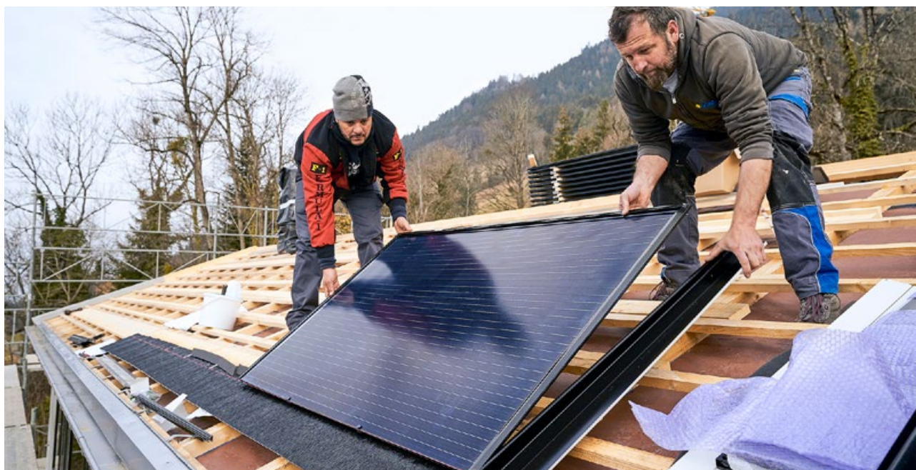
Mounting the lower connector and first row of brackets (see step 7).
