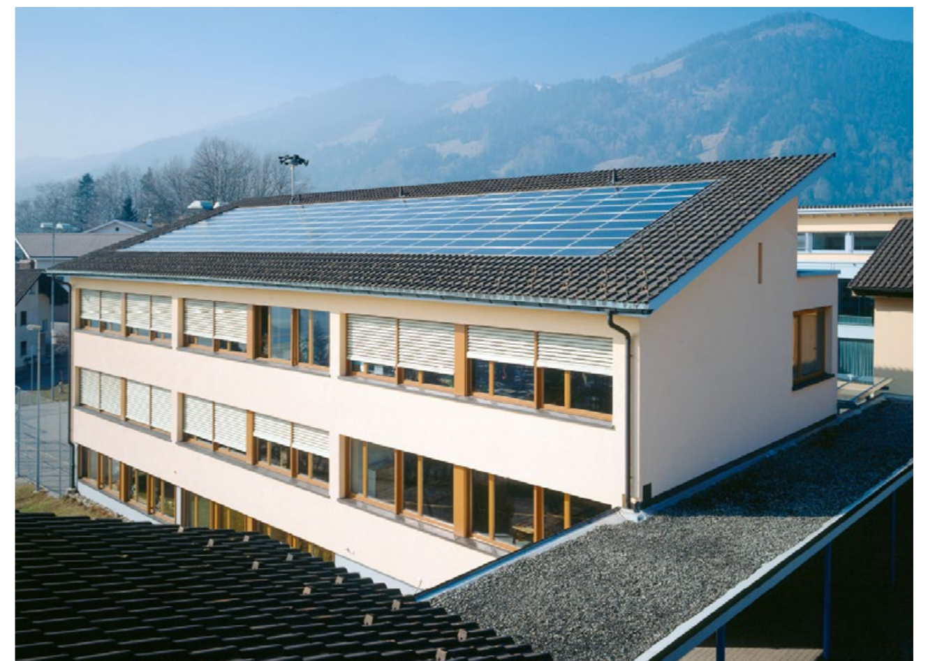
Eggeli school building Sattel (Switzerland)
