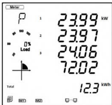
Figure 3-7 Three Phase Power Page
